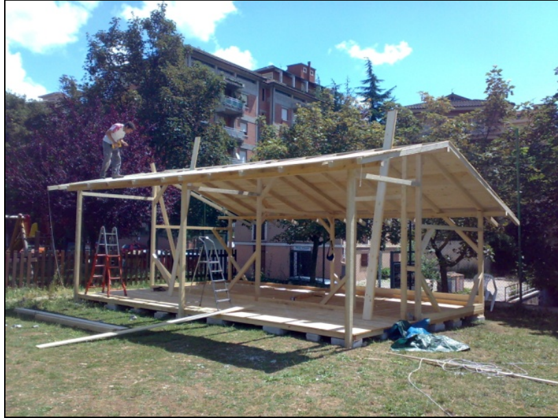
Photo 2. The Media Lab under construction (photo by 3 e 32).
